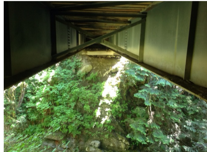
Left Bank Abutment when facing downstream
