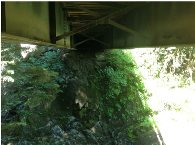
Right Bank Abutment when facing downstream
