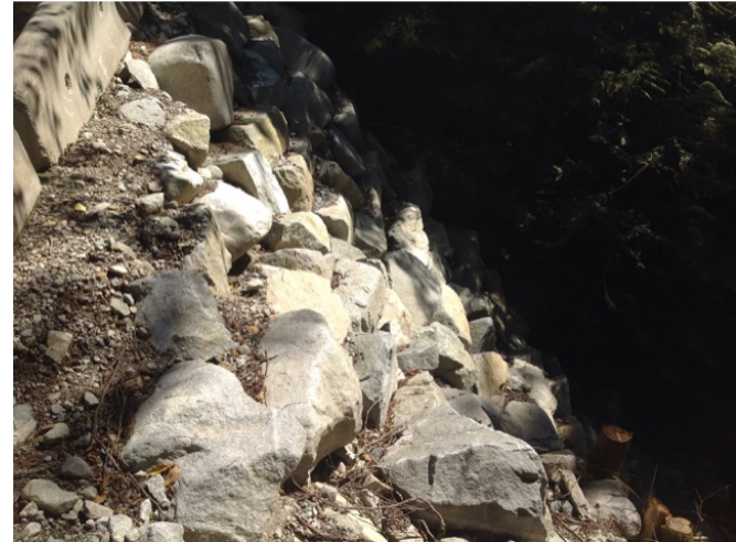
right bank fill slope
